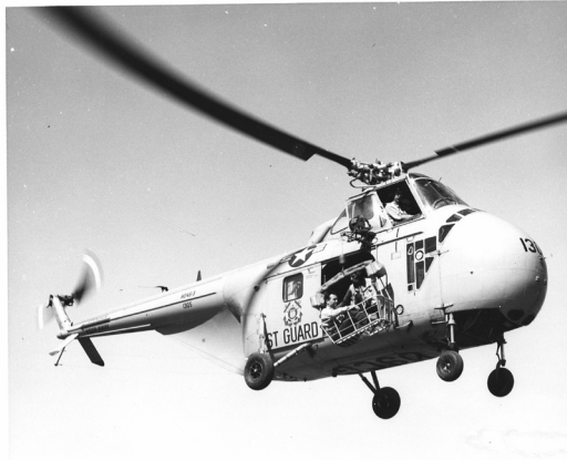
A Sikorsky HO4S (HH-19) Chickasaw based at Air Station San Francisco undertakes a rescue at sea demonstration. Note the hydraulic hoist apparatus capable of lifting up to 600 pounds.
